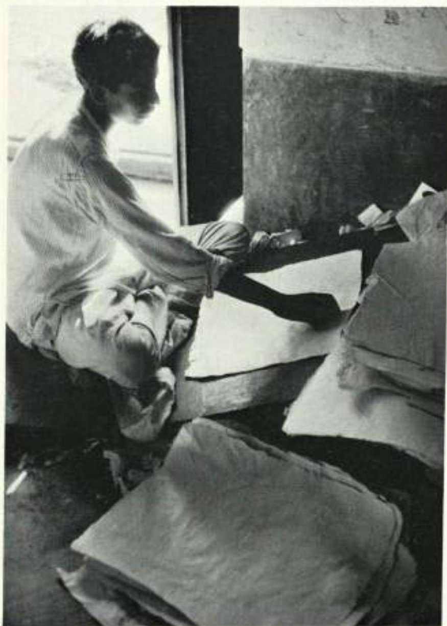
Plate 107. The paper is sized by moistening and dusting with rice or wheat flour. Tripureswar in Kathmandu.
